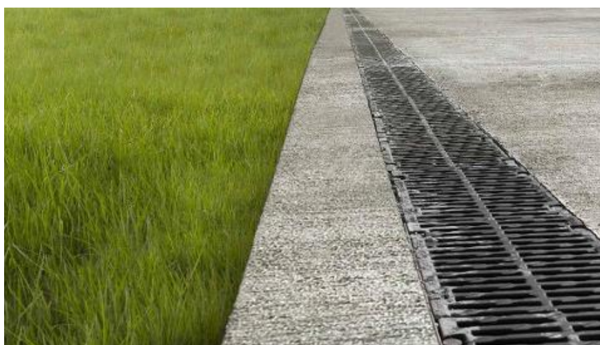
FIGURE 15: SCHEMATIC REPRESENTATION OF STORM WATER DRAIN ALONG THE INTERNAL ROAD
